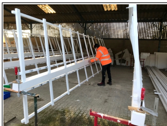
Ready for the shutters
